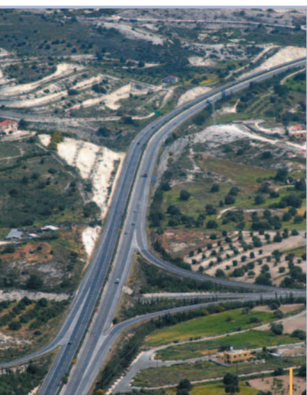
Modern road network, making transport fast, efficient and economical
